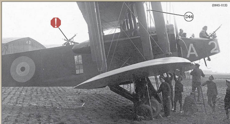
Unidentified late production Handley-Page O/100 "A 2" was photographed on 20 April 1918 and is believed to have been serving with 207 Squadron RAF. Note the twin Lewis guns on Bowen-Williams "Pocket" mountings in the gun cockpit, Holt light on the starboard bottom wing tip, spotlight fixed under the gun turret and partially visible nose art.
