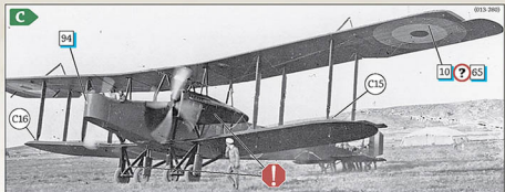
Late production Handley-Page O/100 3124 taxiing on Marsh aerodrome in Mudros Greece on 8 June 1917. Note the very dark gloss painted nacelles, undercarriage struts and full chord cockades and rudder stripes.
